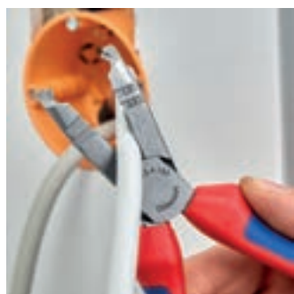
Cutting cable up to Ø 13 mm
